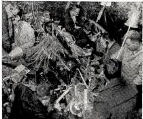
A line crew in the cable pit, painstakingly splicing thousands of wires in one cable to their mates in another.
